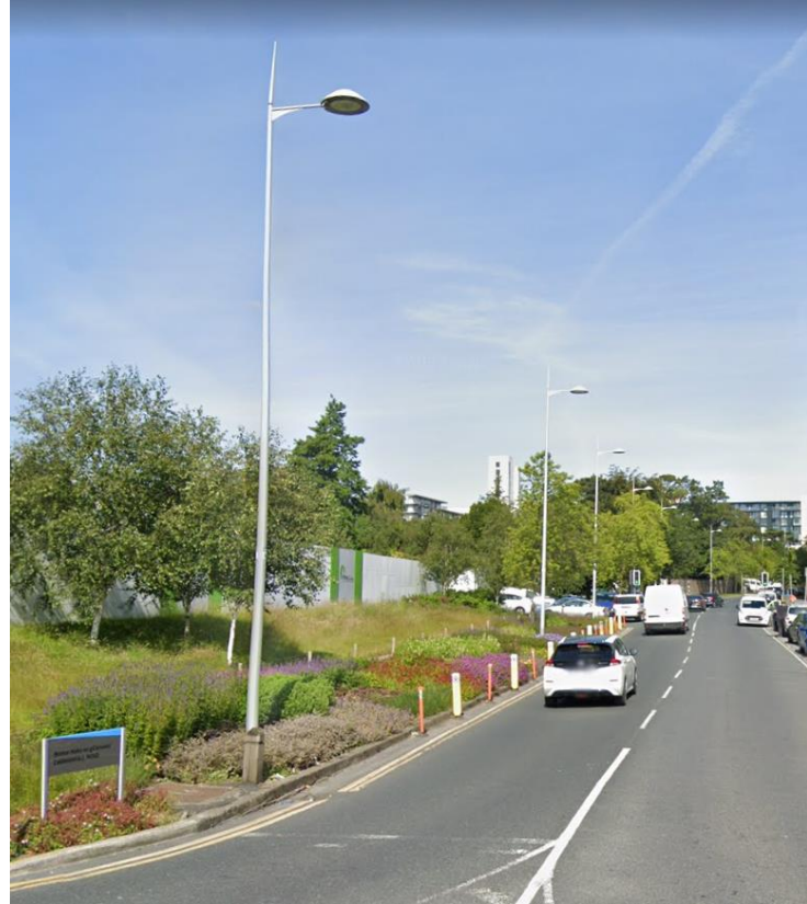
Fig 8.2 Existing DLRCOCO Public Lighting columns on Carmanhall road
